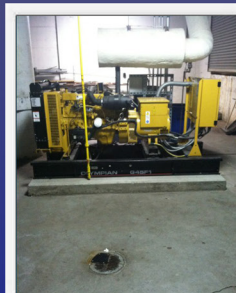
Emergency Generator Upgrade
